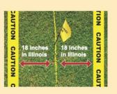
Respecting the tolerance zone protects buried utility lines from damage and also protects you from injury.
